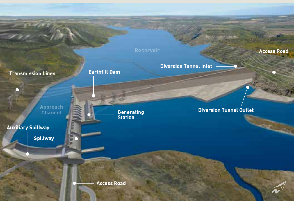
Artist rendering of the proposed Site C dam and generating station (January 2013)
