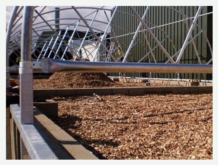
The biogas that is generated from the Anaerobic Digestion will contain H2S and VOC's (volatile organic compounds) which will be sent through two cleaning processes: One scrubbing tower to clean out ammonia; and a second other scrubbing tower to clean H2S before being sent to the biofilter for further reduction.
