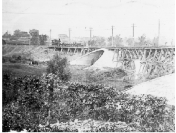
Concrete arch spanning the East Holland River for the Radial Railway.
