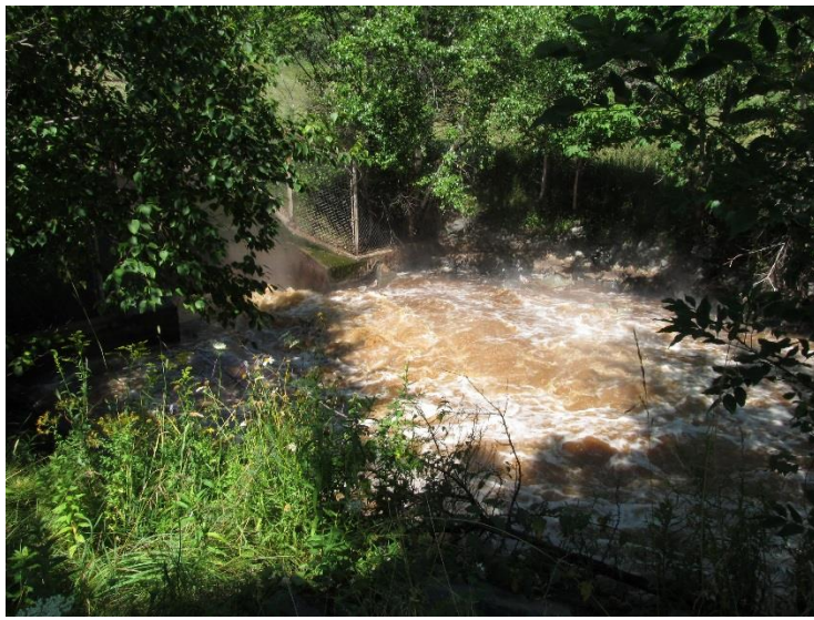
Raw Effluent Discharge, facing northwest
