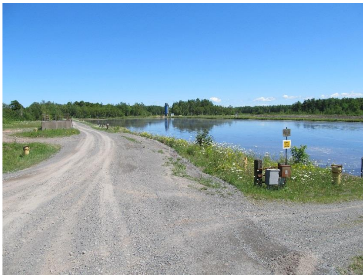
Settling Basins facing southeast from Press Building
