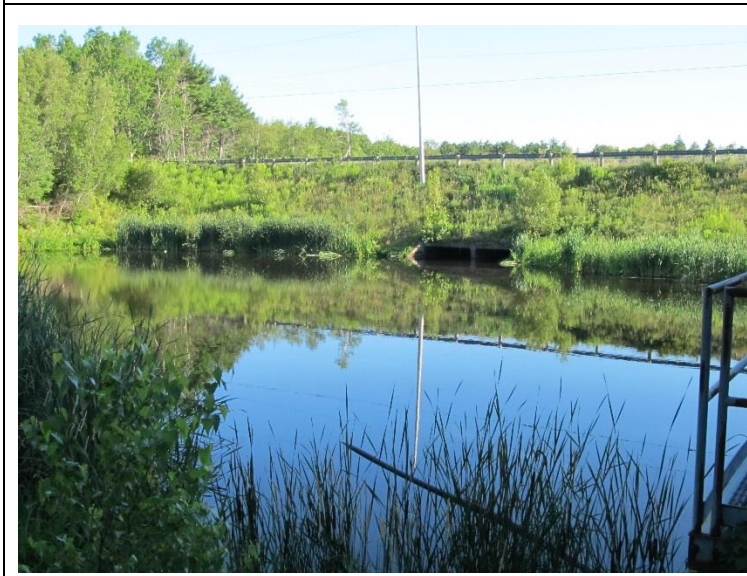
Box culverts below Pictou Landing Road, facing southeast
