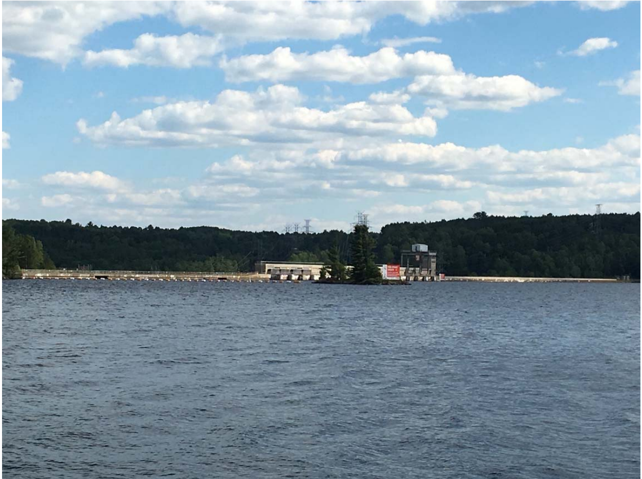
IMAGE 6 – Hydro Dam - OPG's Des Joachims Generating Station from Rapides-des Joachims (August 2016)
