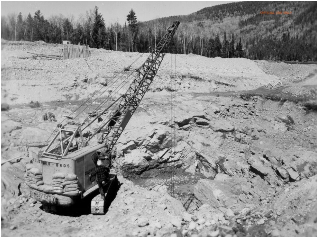
Figure 2.27 Excavation of Bedrock Surface at NPD Powerhouse, Looking North
