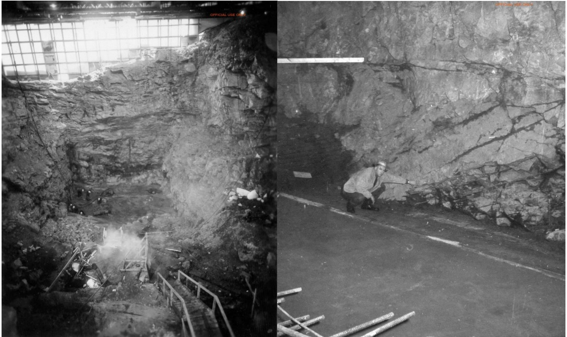
Figure 2.29 NPD Powerhouse Excavations: Left - Looking Northeast, Right – Looking Southeast
