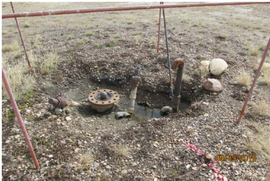
Photo 6: View of the cut and capped Husky Oil Operations Ltd. wellhead at the 14-25 wellsite.
