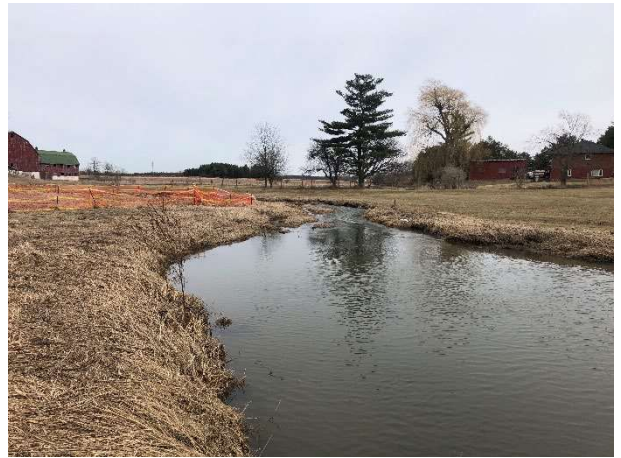
Photo 20: IC-IN Looking Downstream 3/23/2022
