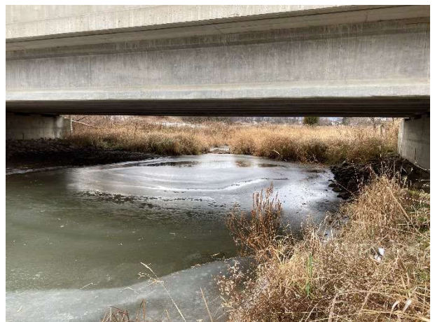
Photo 30: IC-OUT Looking Downstream 11/23/2022
