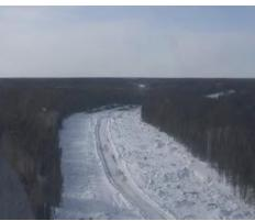
When clearing begins trees are cut down by logging equipment or knocked down by dozers and brush cutters. Salvageable timber is removed and stored for community purposes. Brush limbs and scrap wood are often burned or buried off the right-of-way. The clearing process advances along the right-of-way until completion.
